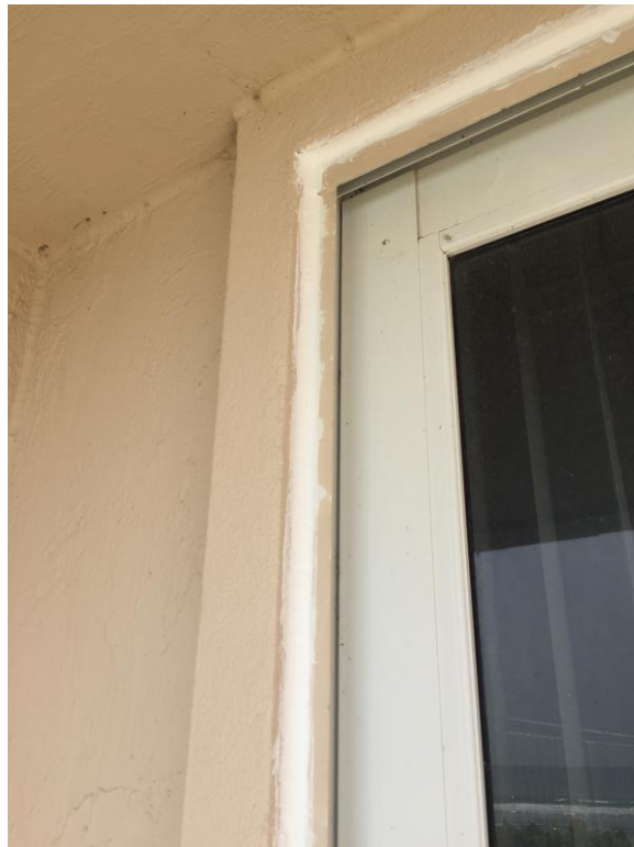
Picture 2: Typical perimeter sealant application
