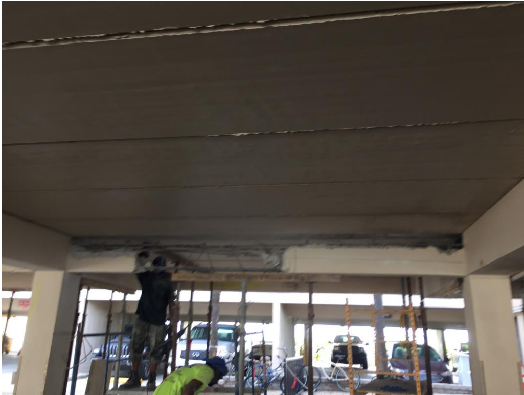
Picture 1: In-progress demolition of lateral transfer beam
